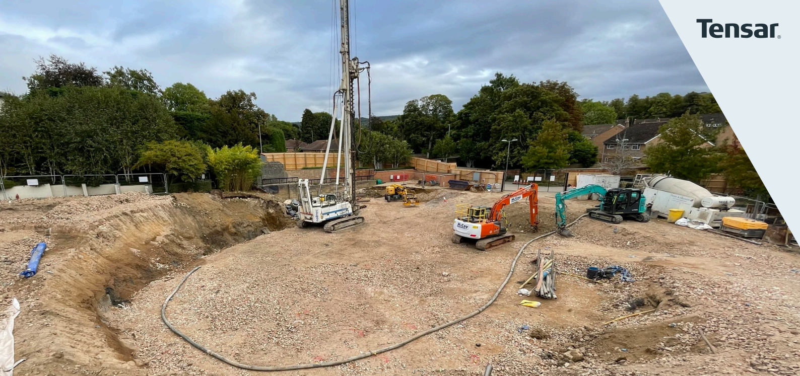
Piling rig in operation on the Tensor Mechanically Stabilised platform
